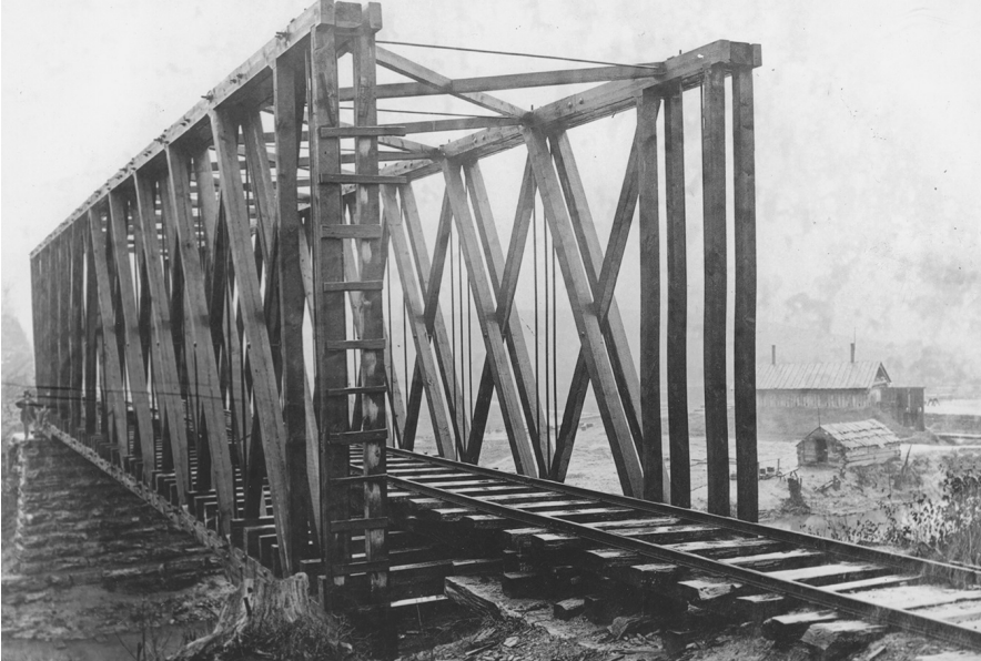
Trace Creek Trestle and Blockhouse, Nashville and Northwestern Railroad near Denver, Tennessee, 1864. Tennessee State Library & Archives
